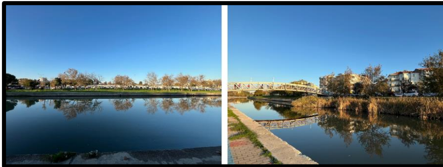
Fig 14. North bank of the river and pedestrian bridge
