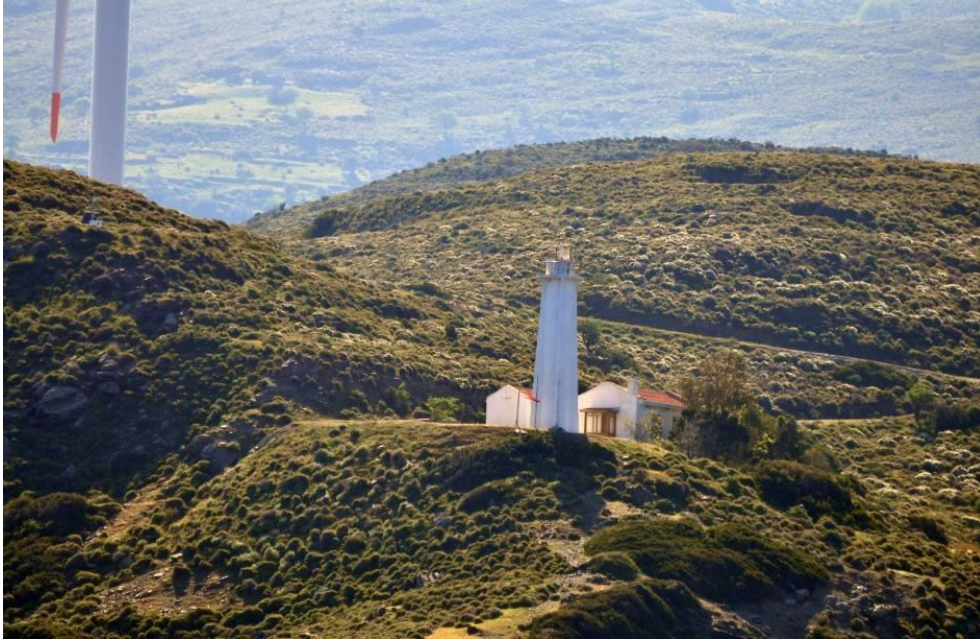
Fig. 6. Sarpıncık Lighthouse and the wind power stations in the background as seen from the sea (Koca Piri Reis Research Ship Archive, 2014)
