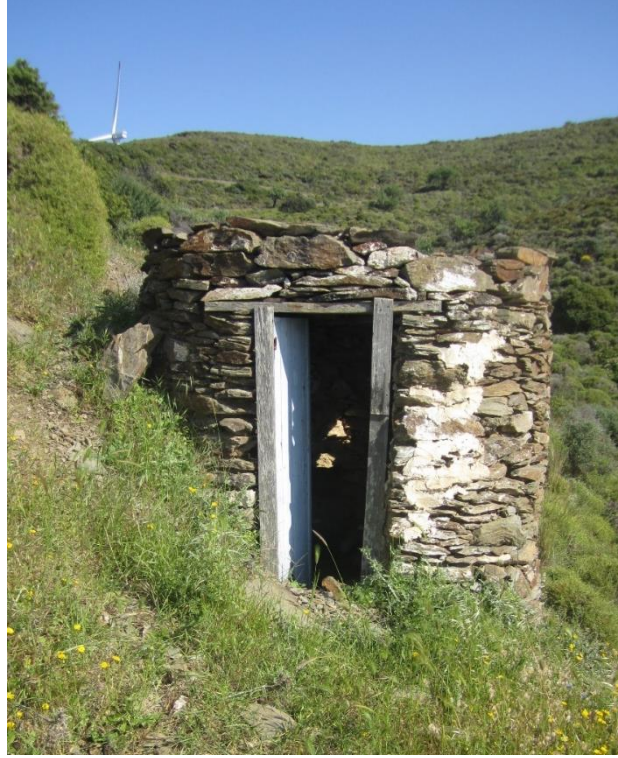
Fig. 5. The local slate masonry, independent toilet of Sarpıncık Lighthouse (O.Basagac Archive, 2014)
