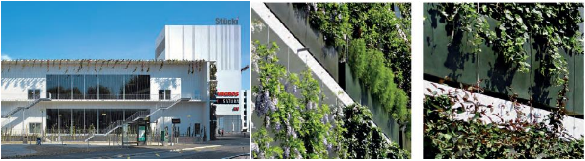
Fig. 5. A shopping center in Basel [12].
