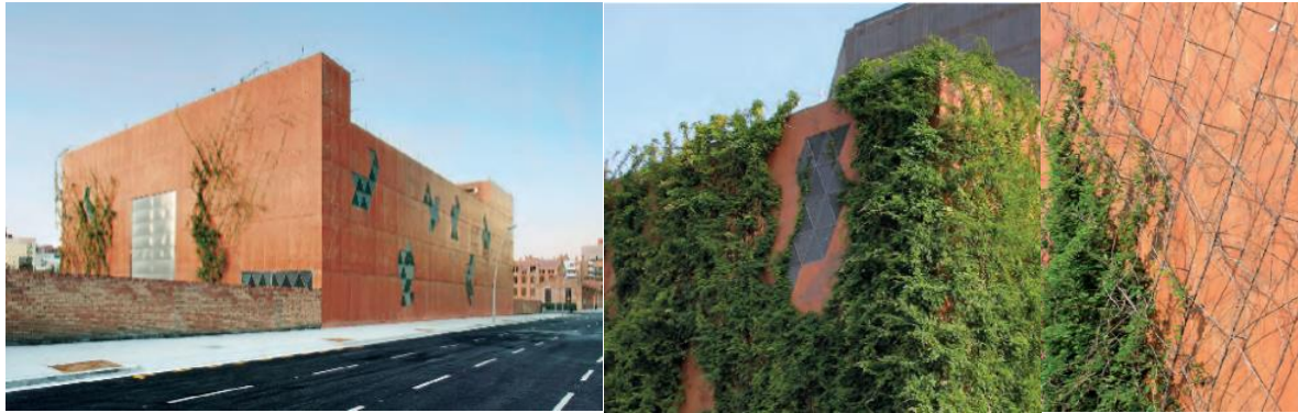
Fig. 3. Transformer substation in Barcelona [12].
